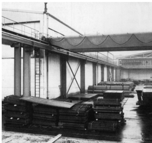
LSV Powerail feeding a steel yard crane
